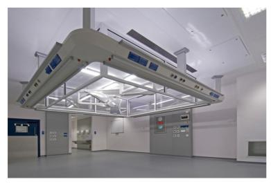
orthopaedic theatre including the installation of a Laminar Flow ventilation system which produces a high purity air supply to reduce bacteria and the risk of post-operative infection.
